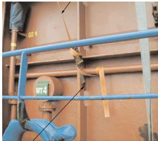
Not a proper securing point
